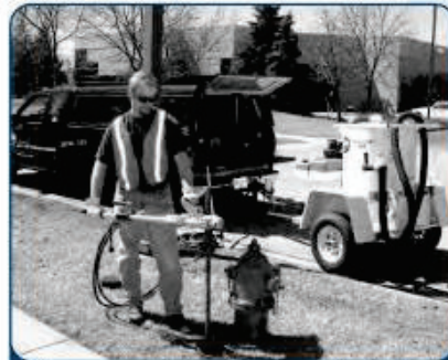
When a water main breaks in the middle of a frigid night, you'll be glad the valves function correctly.
