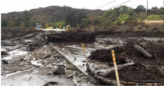
Figure 9: 2018 Debris Flow, Trabuco Canyon
