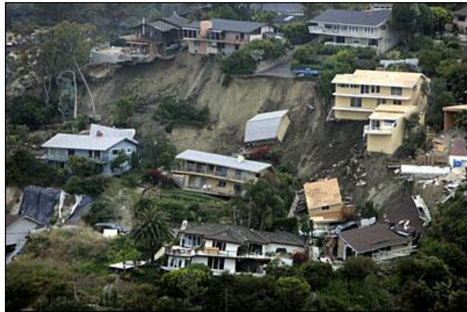
Figure 8: 2005 Blue Bird Canyon landslide, Laguna Beach
