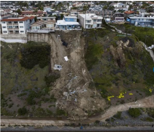
Figure 7: 2023 Buena Vista landslide, San Clemente
