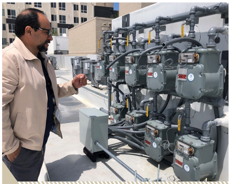
An inspector evaluates a series of vapor submeters at a new apartment development to ensure they are in compliance with registration and accuracy tests before use.
