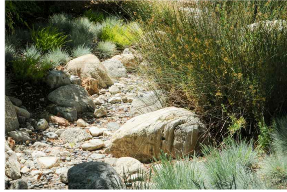
STORMWATER BIOSWALE
