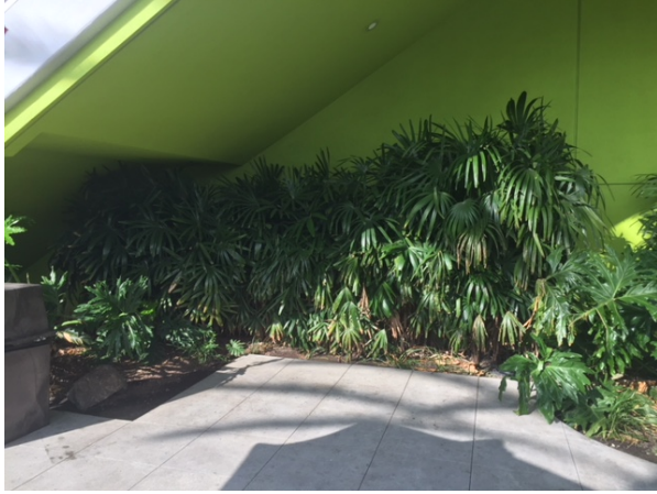
South Wall – W.O.W. Stations
