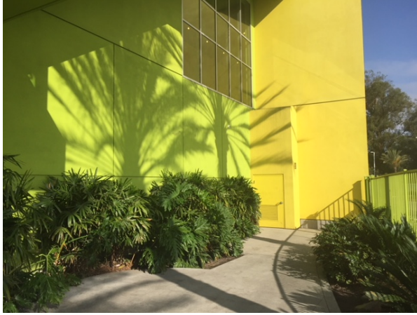
West Corner – Living Wall Area East Side
