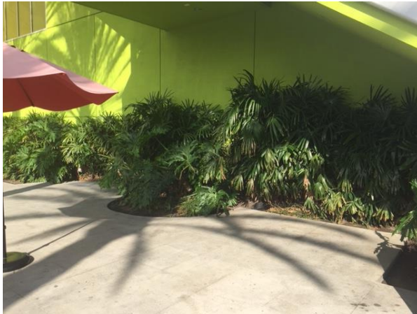
South Wall – W.O.W. Stations West Side Vermicompost
